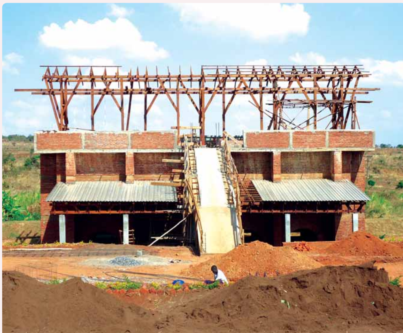
Construction of the Roof of the Kiln
