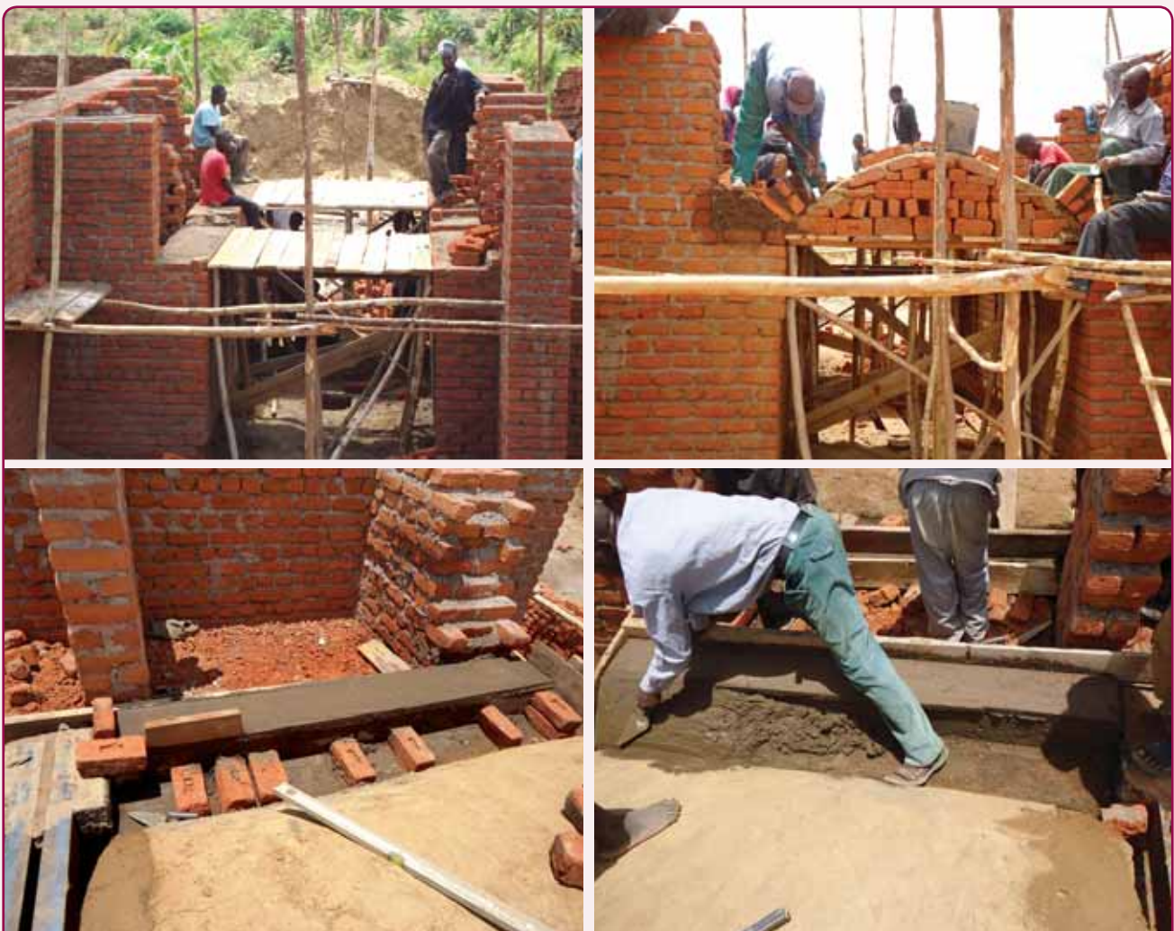
Steps in the Construction of Arch
