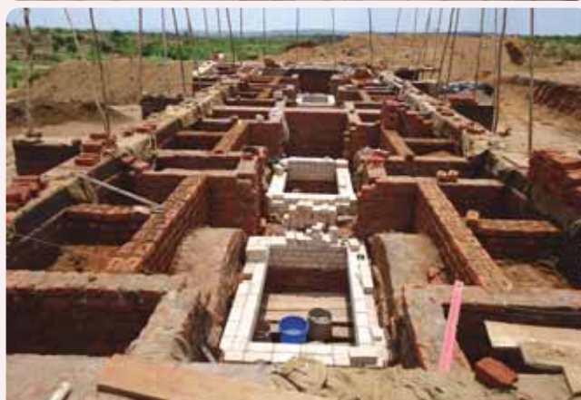
Refractory Brick Shaft Construction
