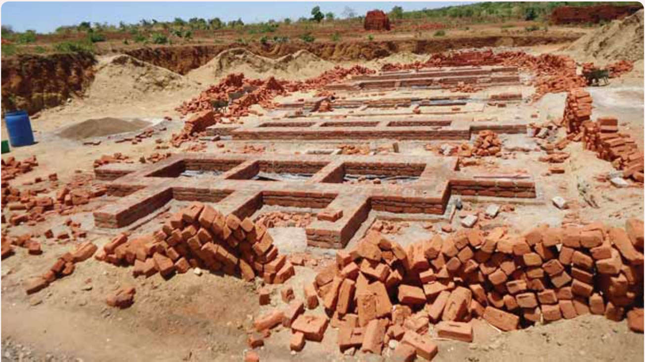
Brick Masonry Work for Foundation
