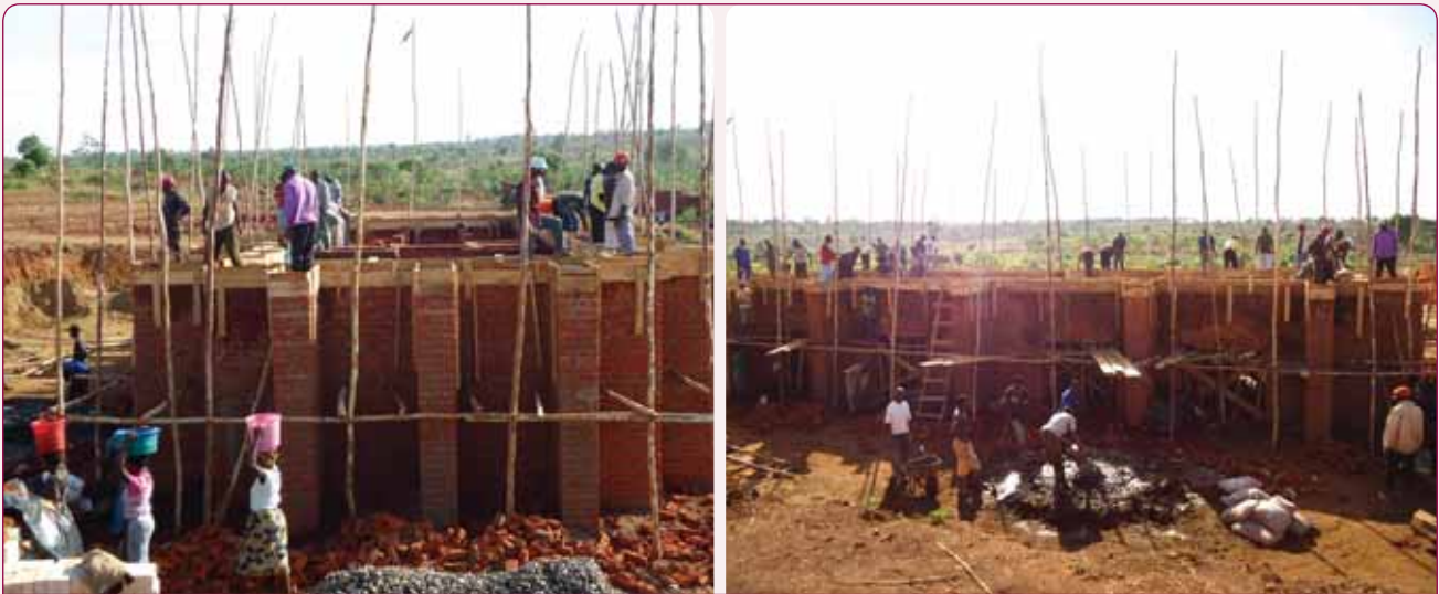
Tie Beam and Corner Wall Reinforcement
