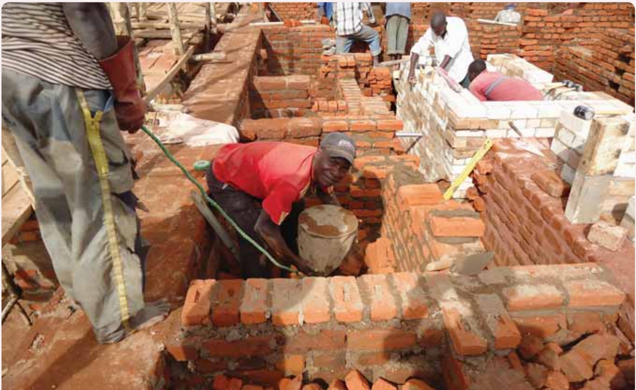
Soil filling work in a VSBK
