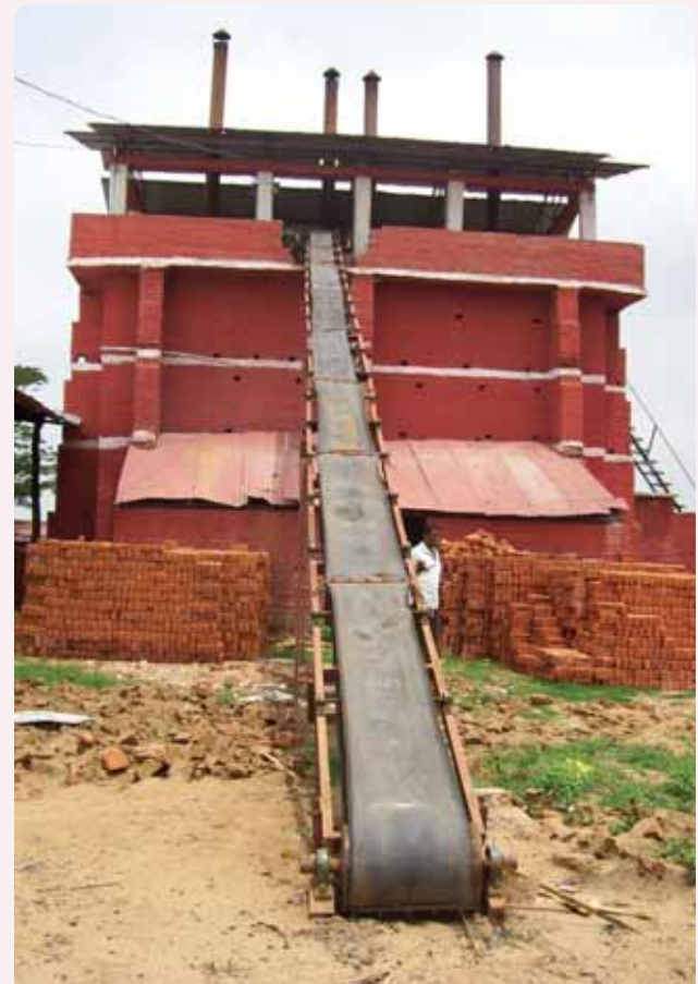
Kiln with a Conveyor Belt
