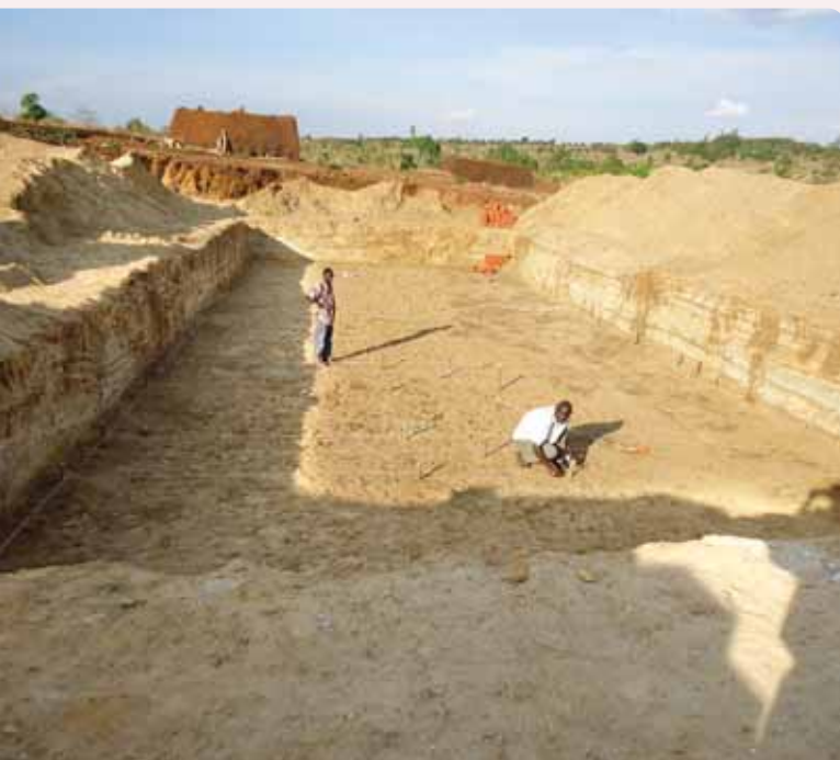
Preparation of Site for the Construction of VSBK
