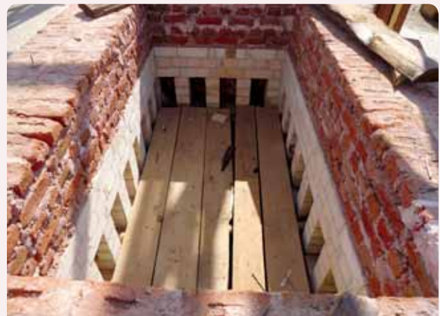
Construction of Upper Flue Duct
