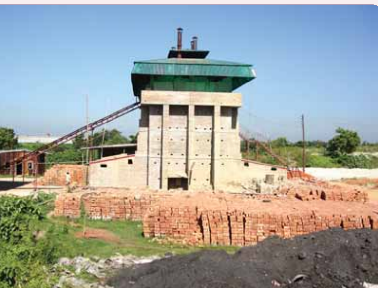
Vertical Shaft Brick Kiln Technology
