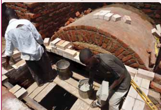
Refractory Brick Shaft Construction
