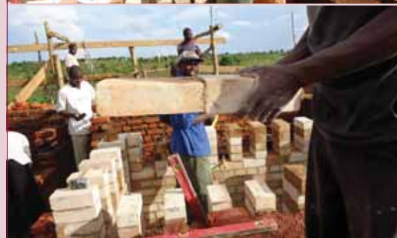
Method of Testing the Quality of Refractory Brick Mortar
