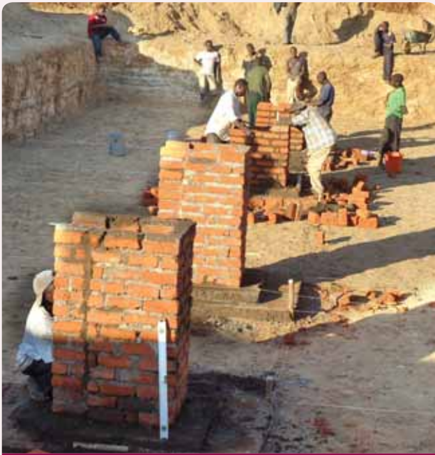
Brick Work for Hydraulic Unloading Device
