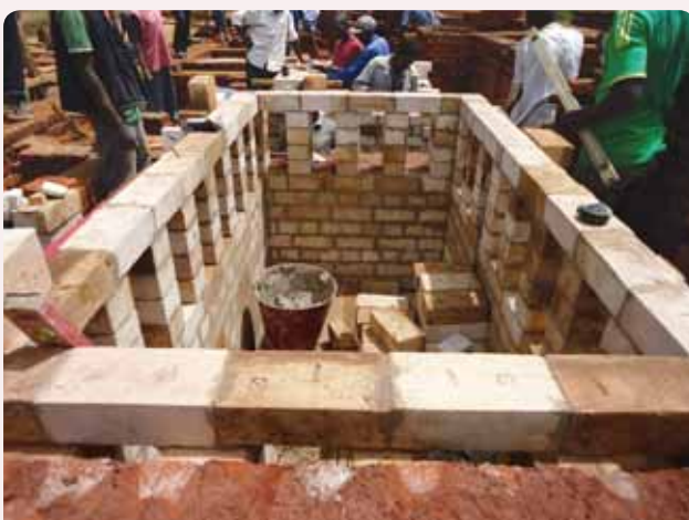
Construction of Lower Flue Duct
