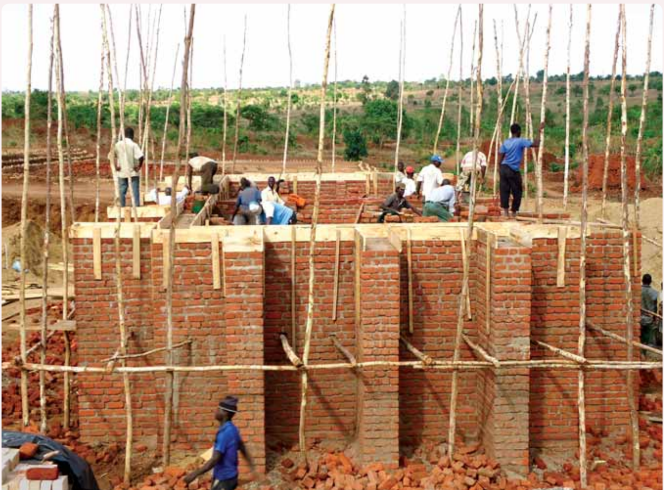
VSBK under Construction
