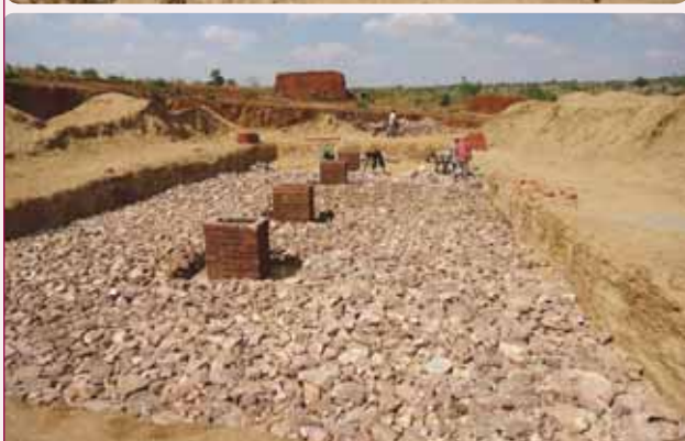
Stone Soling Work for Foundation
