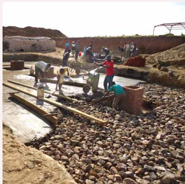
Concrete over Stone Soling
