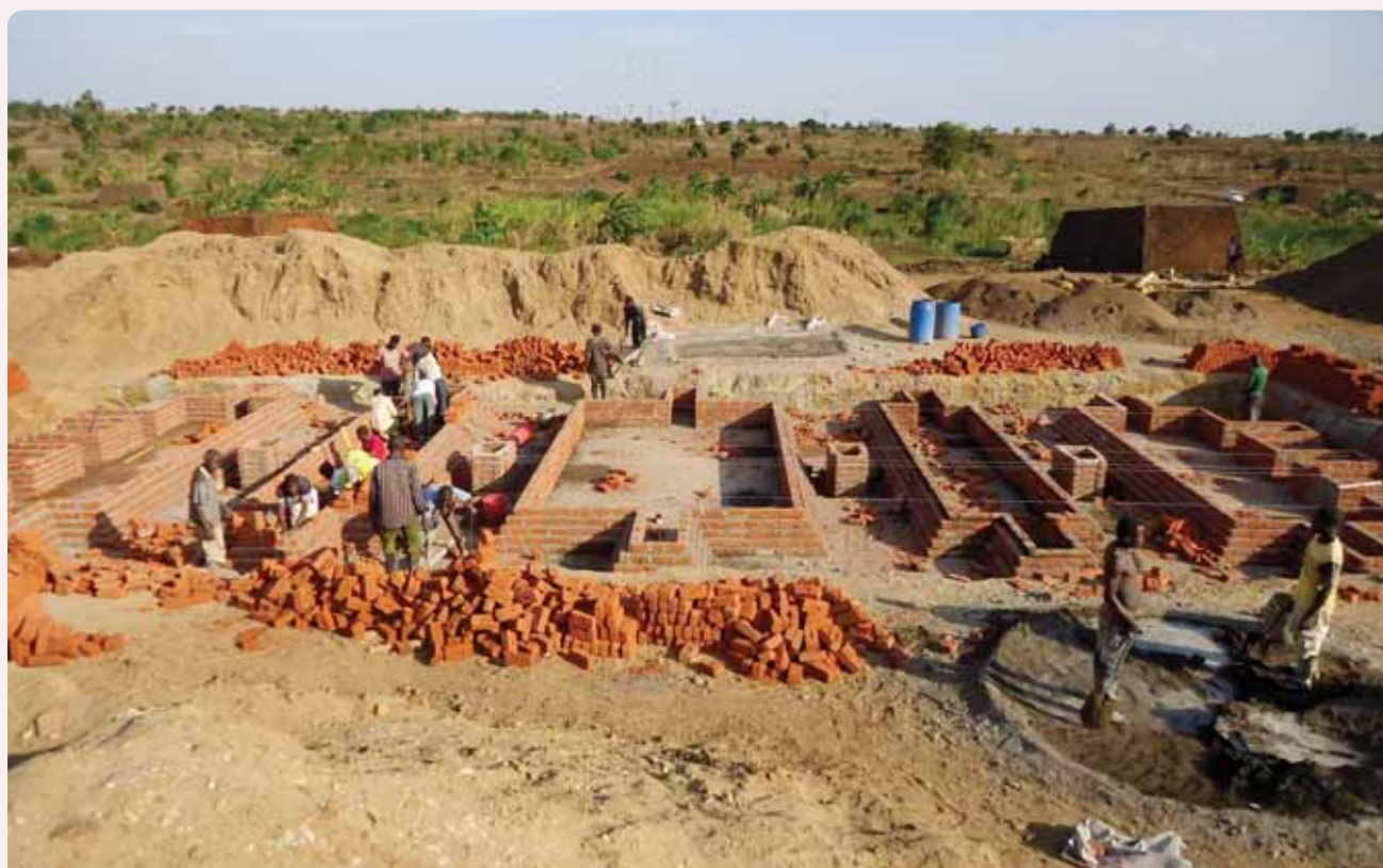
Brick Work above First Corbelling in Progress
