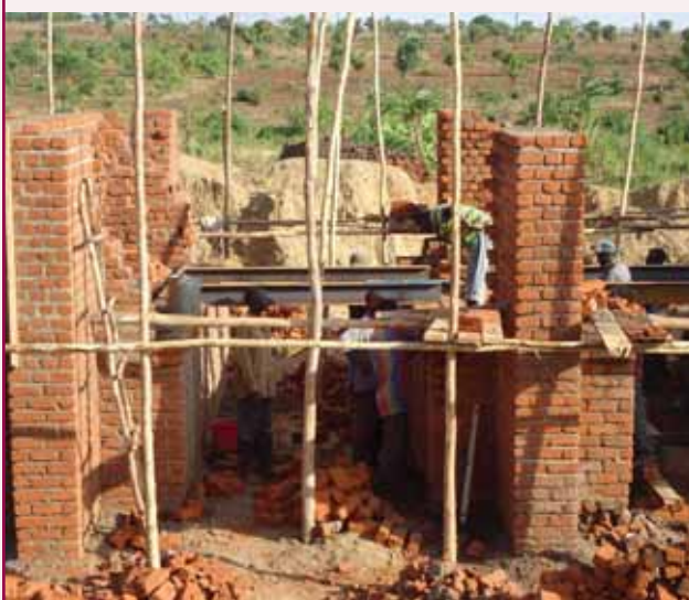
Setting up of I-Beam
